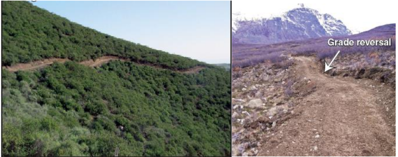
Examples of an OHV trails with reverse-in-grades built in for drainage.
